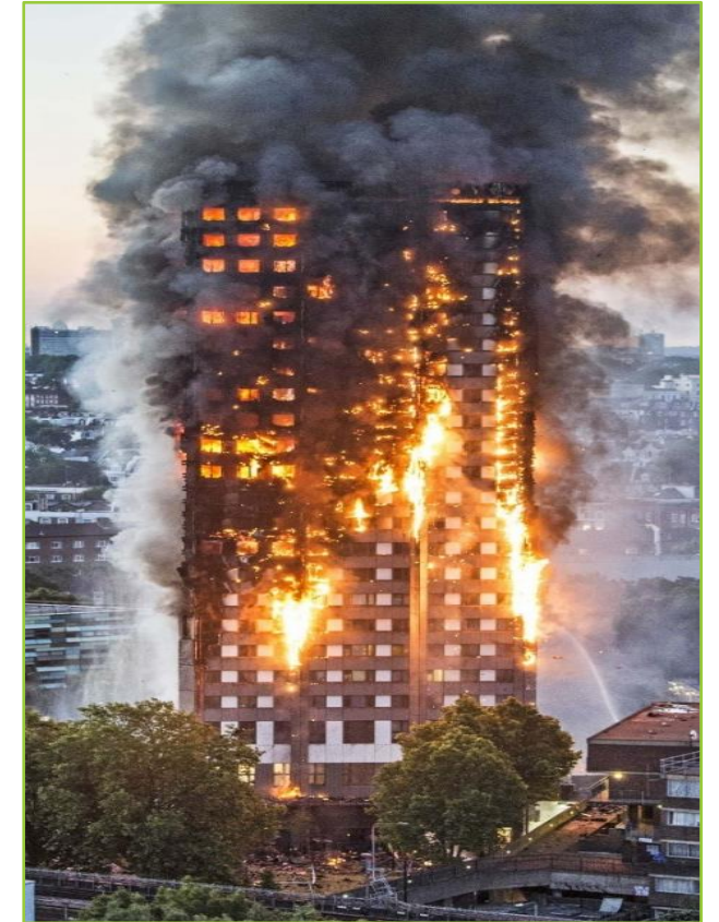
All 24 floors affected by the fire
